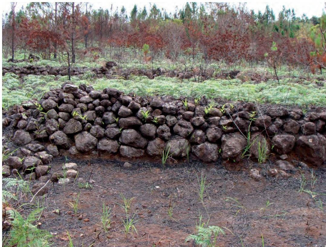
Fig. 7 – Retaining wall constructed as part of a horticultural terrace, site KKR003, Isle of Pines (photo L. Lagarde, 2010).
